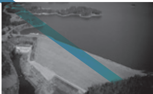
↑ Buford Dam on the Chattahoochee River in northern Georgia, USA. The dam impounds Lake Lanier, 1999 Photo: U.S. Army Corps of Engineers Digital Visual Library Courtesy of Wikimedia Commons
